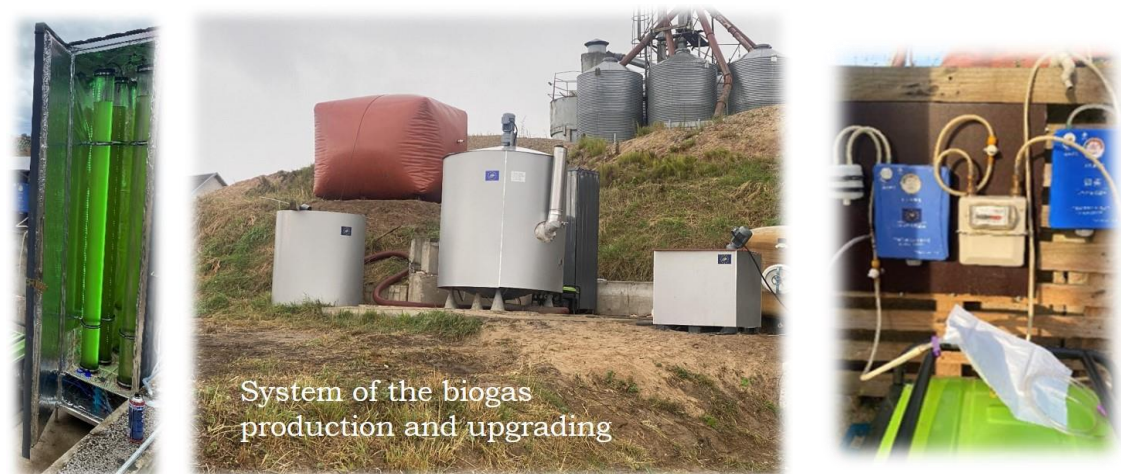
Fig. 6. System for biogas production: images from the left photobiofilter for biogas upgrading, digestate and biogas tank, bioreactor, biomass shredder, control panel and generator.
